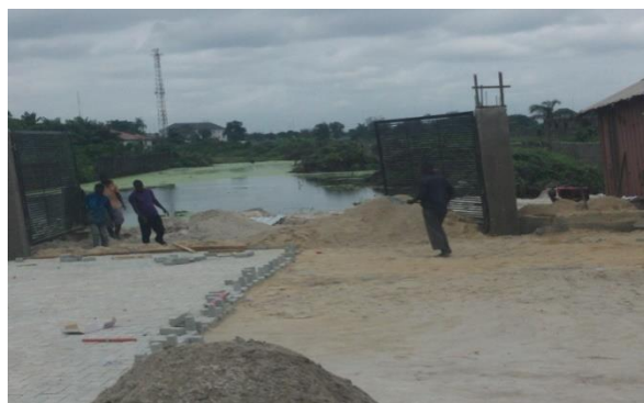
Plate 3: Sand filling
